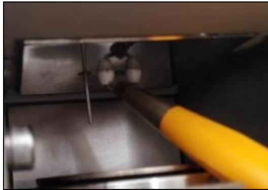
Figure 3: Cleaning Ignition Device Surface
